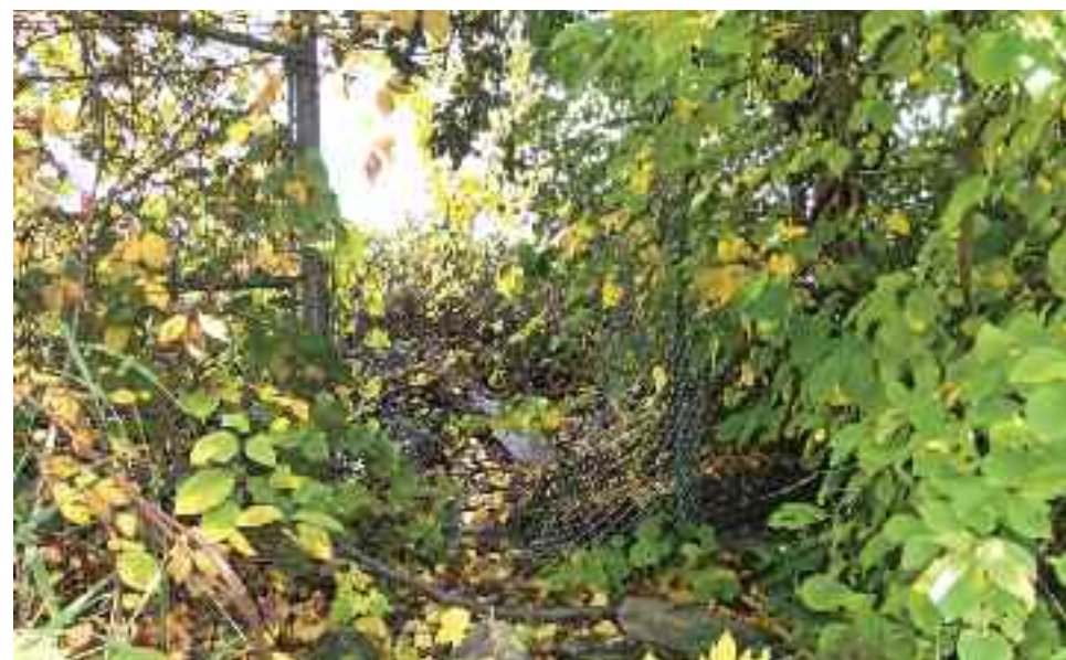
This image shows where the fence dividing a private property from the railroad tracks was cut. Public Works is repairing in an attempt to keep the coyotes out.
